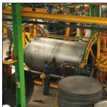
Assembling the tank sections, front and rear walls
